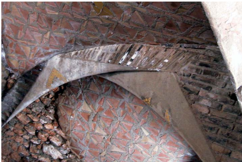
Fig 9. Hyperbolic paraboloids meeting on their directrices at the Colònia Güell Crypt
